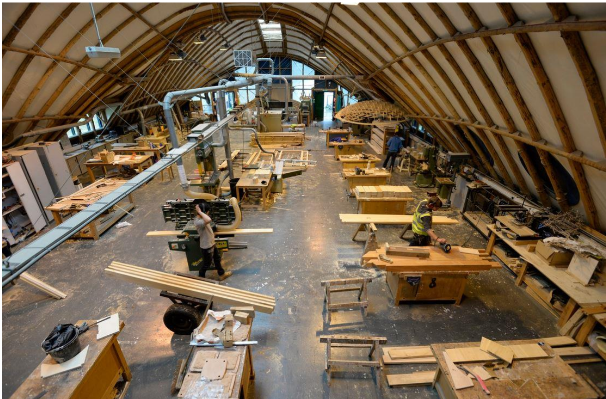
Photo 6 The Workshop at Hook Park, build out of elastic pole stage thinning's (picture website Hook Park)
