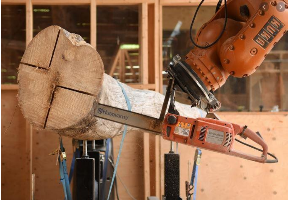
Photo 7 Robotic milling at Hook Park (source Jeremy Ralph)
